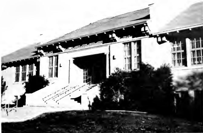
Photo 6. Morningside Elementary School. Rehabilitated to meet the requirements of the Field Act.
